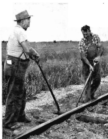
Ganger A. E. Rosenow (left) and Repairer A. J. Davis are packing the track near Rochester.
