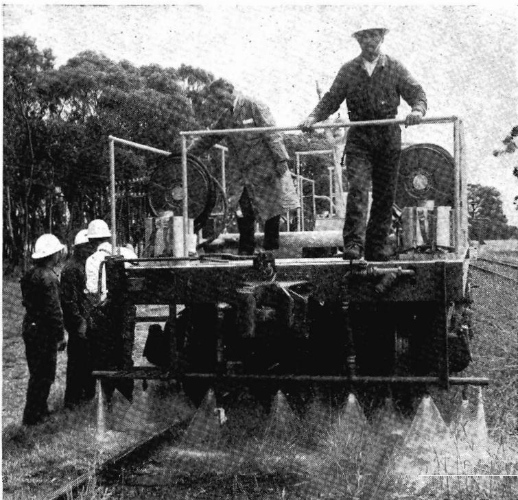
Water boom at front of wagon extinguishes fires in sleepers.
