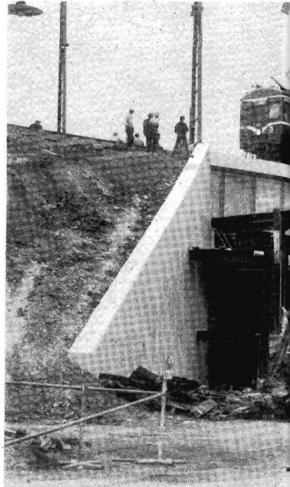
The week-end of August 2 and 3 saw completion of a further stage of the reconstruction of the Swanston Street bridge over the railway lines near Flinders Street station. While the bridge was closed to traffic, old girders, varying from 10 ft. to 44 ft. span, were replaced with new ones. The picture shows a section of old girder and roadway being lifted out.
