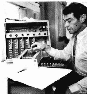
Lighting and Power Design Engineer, Don Rowe, indicates the PROM memory banks inside the brain box of the electronic train destination board controller. The memory banks control the five output switching cards in the control box behind Mr. Rowe's hand.
