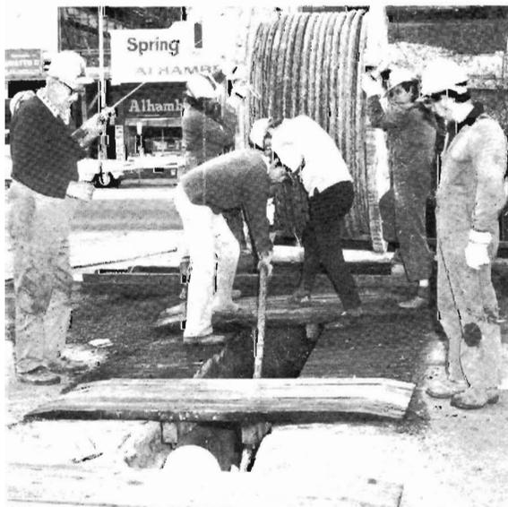
Not gold mining, not tunnelling into trouble (or a bank vault), just feeding a new 6,600v power cable under Spencer Street terminal.
