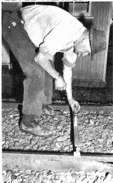
A lot of back breaking work has gone out of track maintenance since mechanised maintenance was stepped up, but there's still plenty of opportunity to bend the back! Caught by the *Rail Ways* camera was Special Ganger Ted Wyatt checking the cant (superelevation) on the standard gauge line curve through Bowser, 6 km (3½ miles) from Wangaratta. Track machines had been working on the line and Ted was checking that the 102 mm (4 in.) cant was correctly aligned.
