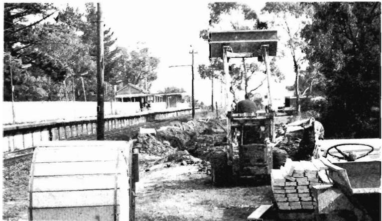
Doesn't look much like the way to bring a better train service to the Lilydale line . . . but it is. Into a trench being dug will go the power cable for a new signalling system between Ringwood and Croydon to allow closer spacing of trains and reduce delays. Work should be finished by November.
