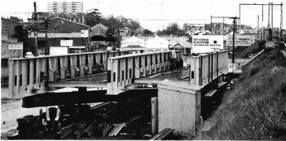
*Bridge No.2*, City Road Melbourne, where the pre-fabricated bridge structure is being moved by rail bogies prior to position. (Details of this particular project were outlined in January's *News Letter*. The job was delayed for about six weeks because of difficulties in moving the steelwork.
