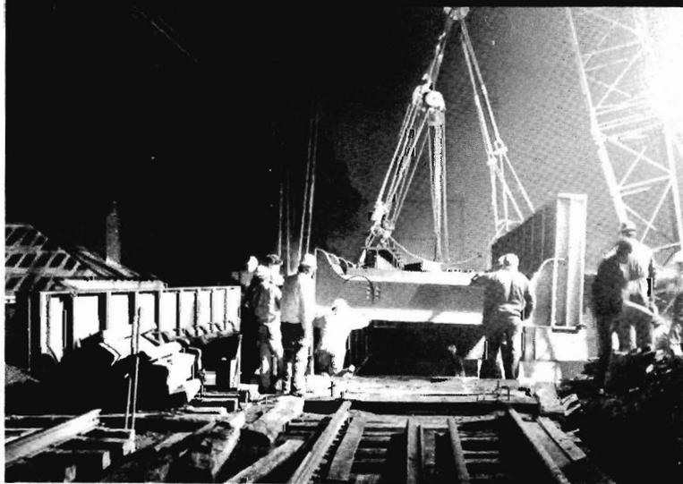
Bridge building was big news during July. In another week-end battle against fog and time, railway workmen positioned a pre-fabricated steel bridge structure at Francis Street, Yarraville. During the early hours of the morning, when the fog lifted a little, this was the scene as workmen guided the bridge into position.
