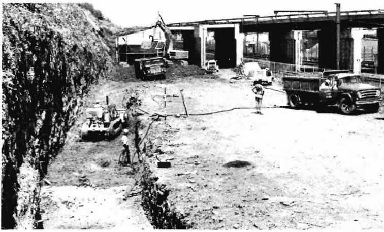
Preliminary work for a retaining wall at North Melbourne has already been completed and scaffolding erected for initial work on driving a new opening through the flyover.
