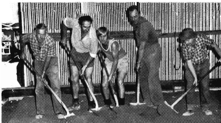
Surfacing of the loading ramp in the Wodonga goods shed nears completion as the local works gang spreads a sand base in preparation for the final cementing. The gang, from left to right, is J. Muir, E. Coulston, R. Jackson, B. Waugh, and J. Kowalczyk.
