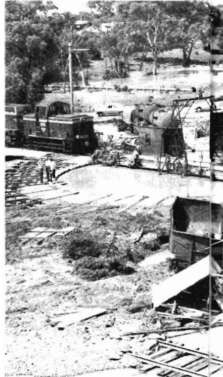
WORST HIT AREA was the locomotive depot of water swept through, flooding the turntable pit, derailing wagons, damaging buildings, and carrying away the foreman's office.
