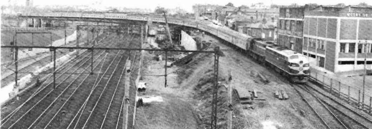
At North Melbourne, the retaining wall alongside the flyover has been completed as has the base of the ramp. *Southern Aurora* can be seen going over the new opening in the flyover. The approach ramp on the other side of the flyover is also completed.
