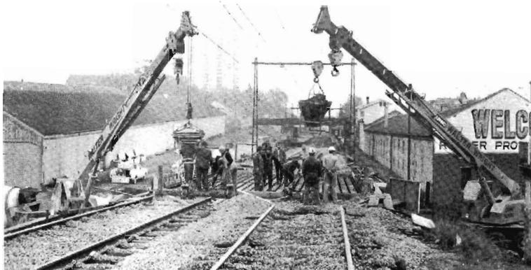
While the St. Kilda line was out of action last month for renewing the City Road bridge, railway workmen also took the opportunity to do a similar—but smaller—renewal at nearby York Street bridge. Here, in 16 hours, new beams and decking replaced the old, concrete was poured and the tracks restored, to give the old bridge a new lease of life.
