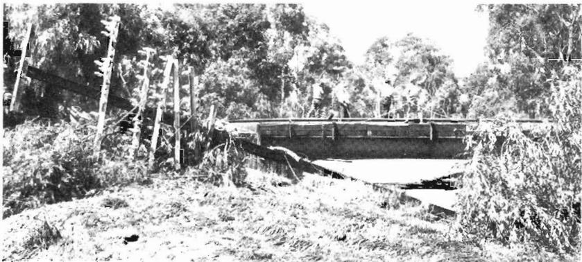
COMMUNICATIONS WERE CUT when four poles were washed out. The poles carried communications and signals power and circuits. Emergency arrangements to keep trains running in the unaffected areas were achieved by using P.M.G. telephone circuits and local S.E.C. power.
