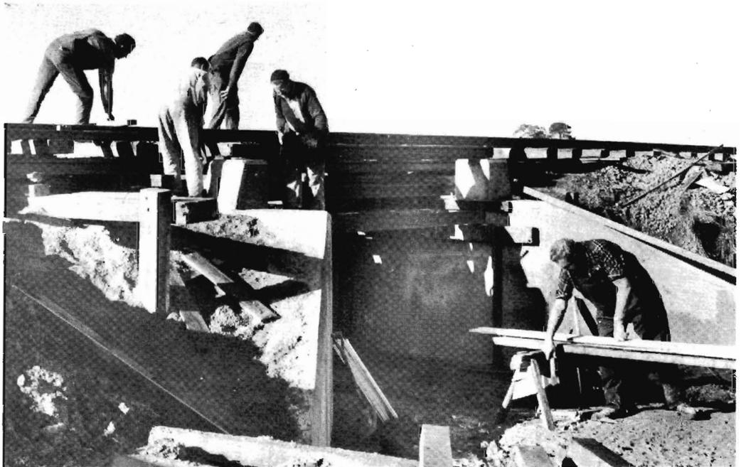
**LITTLE BRIDGES** are also part of the railway scene. Here, at Myamyn, workmen are busy lining up a small concrete culvert.
