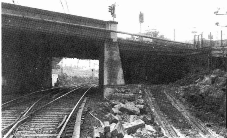
Progress on the Footscray quadruplication is now centred on approaches to the Hopkins Street bridge. On the Williamstown line side (above), the bridge approach has been prepared, while on the St. Albans line side, workmen are blasting their way through the bluestone. Space for one of the tracks from South Kensington has also been finished and the embankment sprayed with concrete to stabilise it. Work will start soon on cutting the way for the track to come through on the south side.
