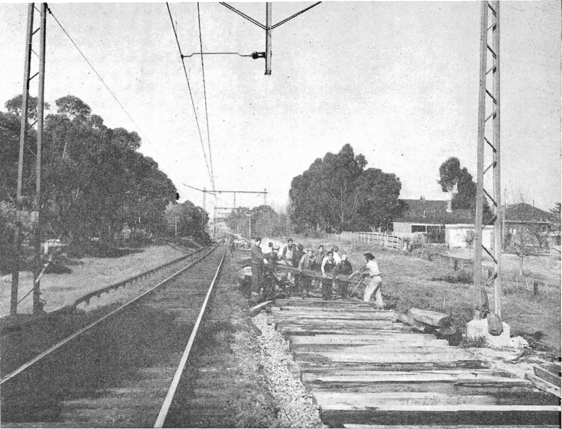
Laying New Suburban Track
