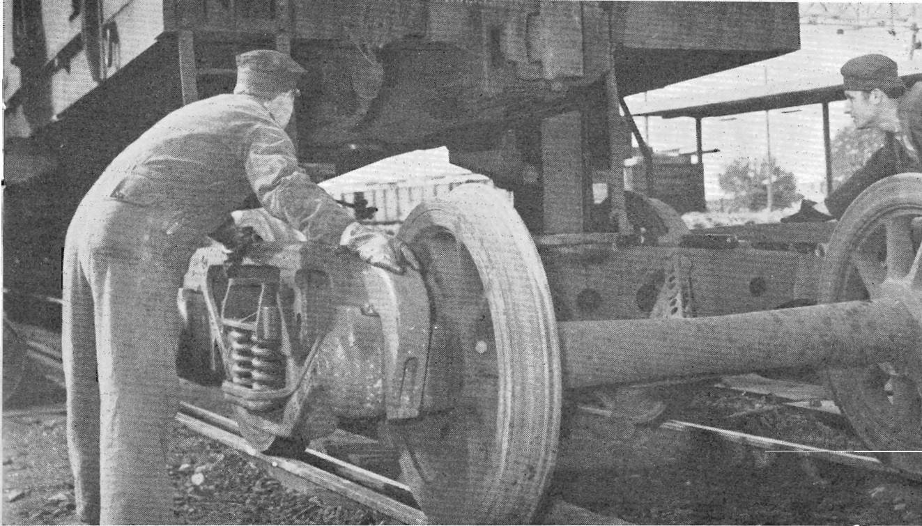
CHANGING THE BOGIE UNDER A 50-TON LOADED WAGON
