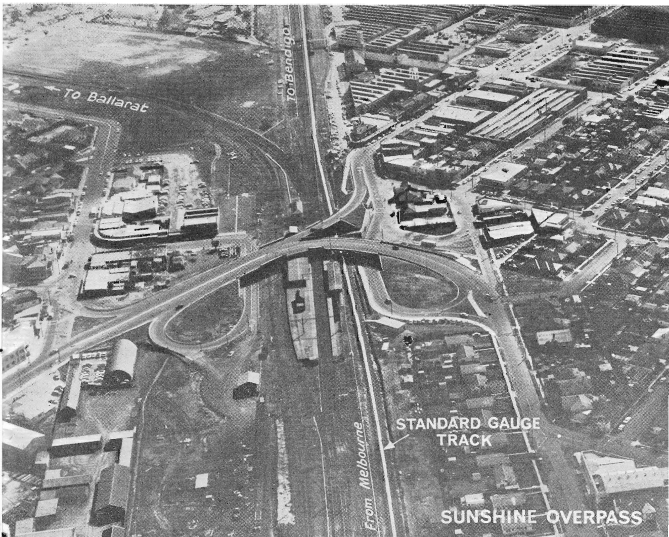
AN AERIAL VIEW OF SUNSHINE OVERPASS
